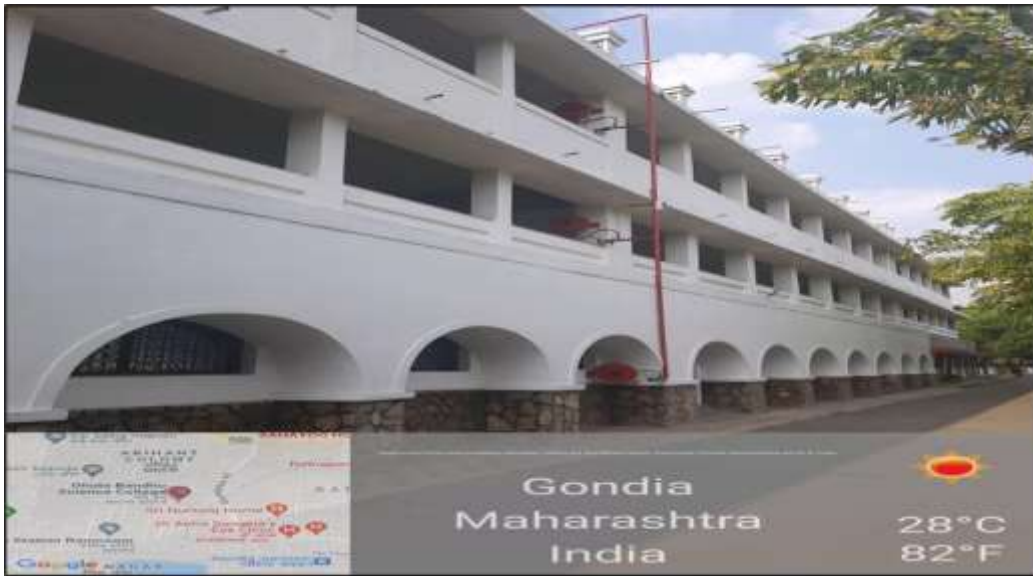
Fire down comer riser system
